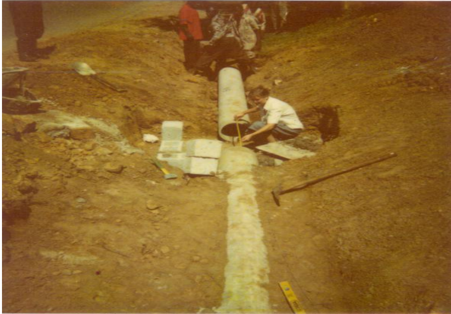
Ms. Stephanie Bache on a construction Site
