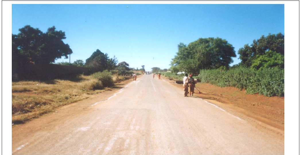
Road construction works set to pick, under RoadSIP II
