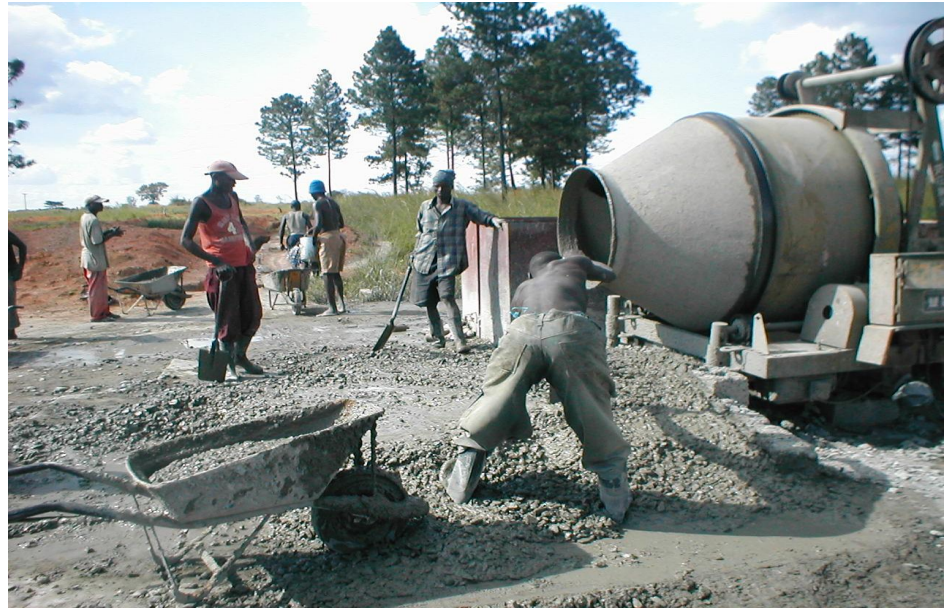
Construction activities have continued to increase over the years
