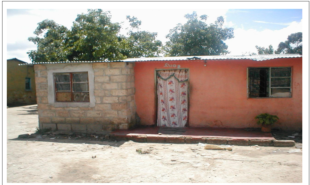
Some middle class workers are now living in informal housing units or in servants quarters
