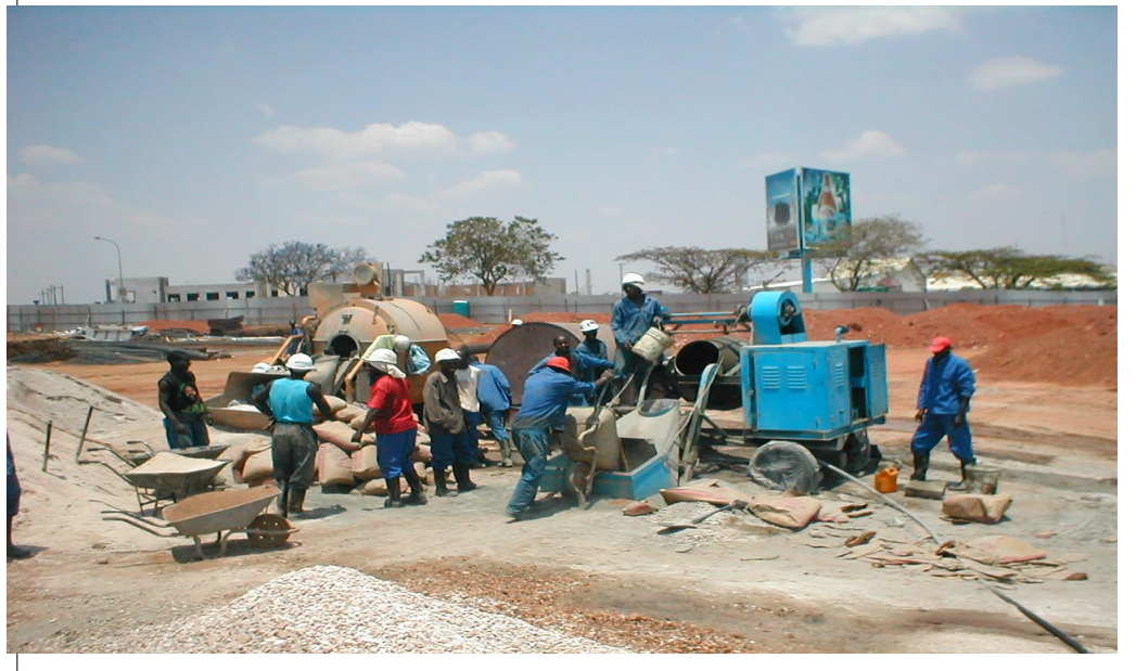
Private Sector Works in progress—Private sector construction workers busy at work.
