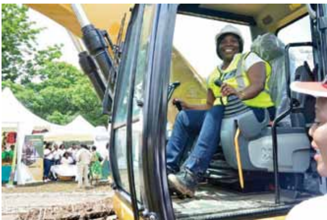
NCC Showcasing Excavator operation during International Women's Day commemoration in Lusaka at the Showgrounds.
