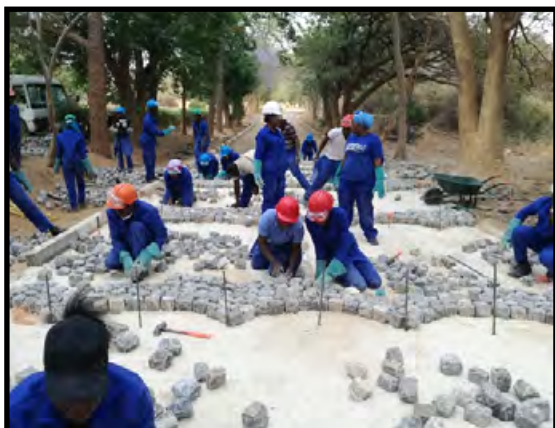
Segmental arch pattern under construction
