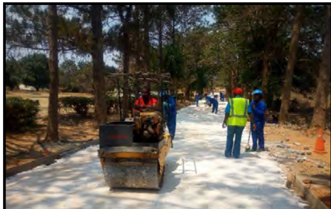
Final paved layer being compacted
