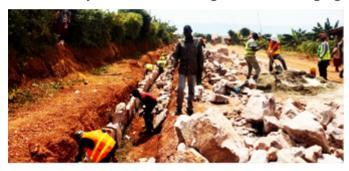
contractor had a 14.2km of road, and had employed 52 workers from the area of construction. The scope included pothole patching, desilting of side drains and culverts, vegetation control as well as debris removal and other maintenance needs such as clearing embankment sections, debris removal from bridge openings and small landslides that may occur along the road. These contractors are contracted on previously rehabilitated road sections to ensure they keep them in maintainable state.
